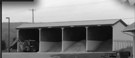
Salt/Dry Bulk Sheds
